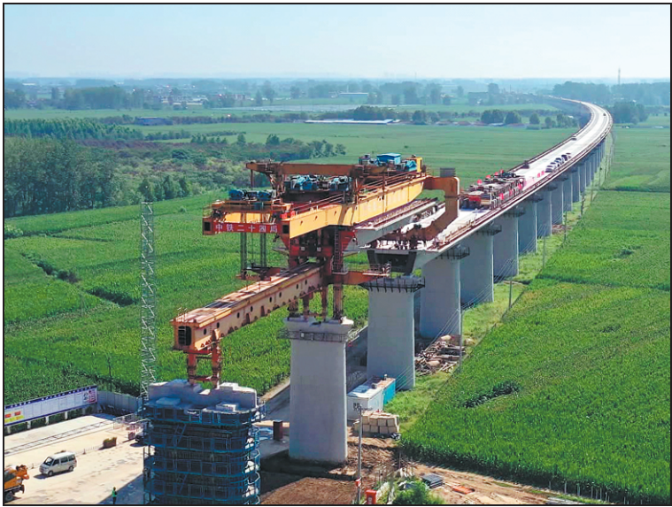
A recent drone image captures the ongoing construction of a bridge along the Fuyang-Huaibei High-Speed Railway, which will soon connect three previously unserved counties in Anhui province. China Railway Construction Corp's 24th bureau reported that it successfully placed the final 700-metric-ton box girder in a significant 799-girder project. This milestone marks a crucial step toward the railway's full connection, signaling massive progress in boosting integrated development of the region. PROVIDED TO CHINA DAILY
