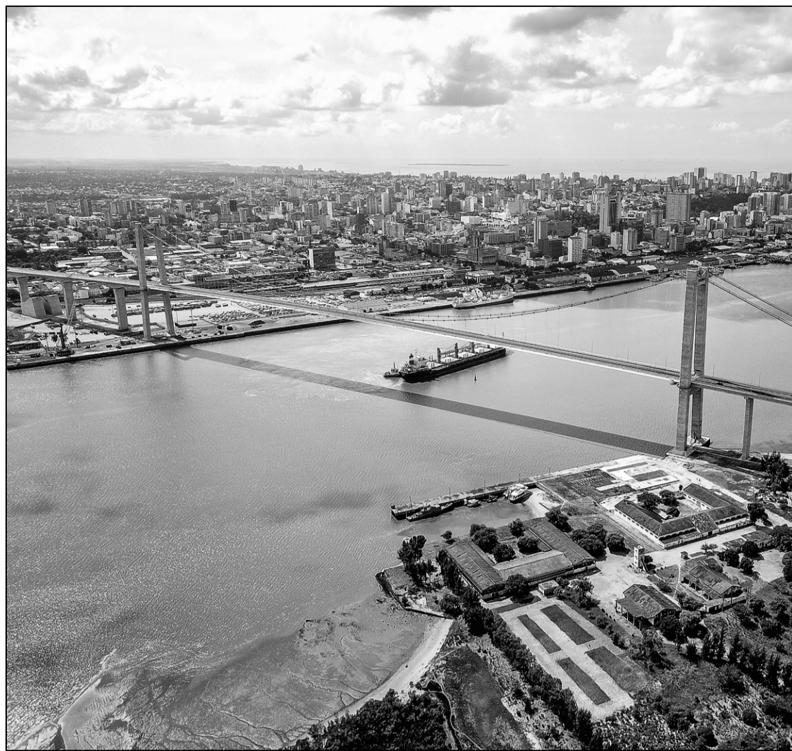
The Maputo-Katembe Bridge in Maputo, Mozambique's capital, in 2019. The bridge, which was opened in 2018, applied China's highway standards. ZHANG YU / XINHUA
